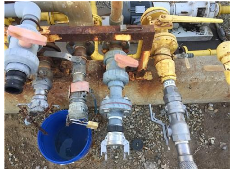
Chemical unloading operations at the time of the incident (Source: CSB / MGPI)
